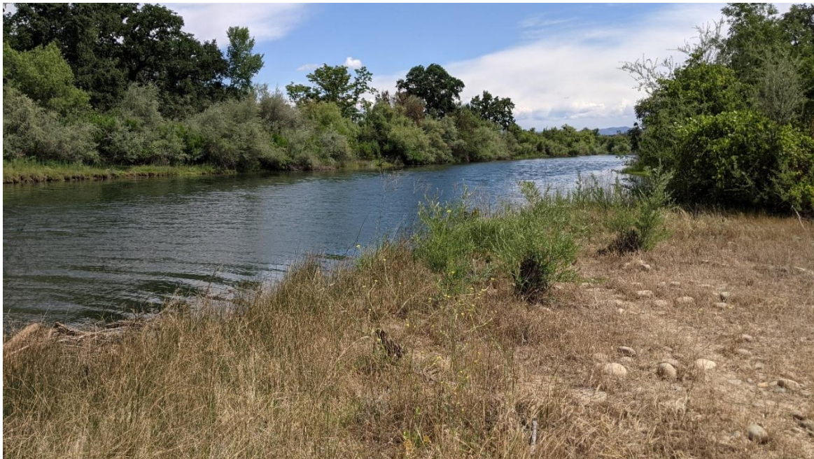
Figure 10. Photopoint 5b. PPT 5 faces northwest and is located on the left bank at the old bridge abutment. Photo shows the river just upstream of the bridge abutment and portion of river where submerged I-beams are located.
