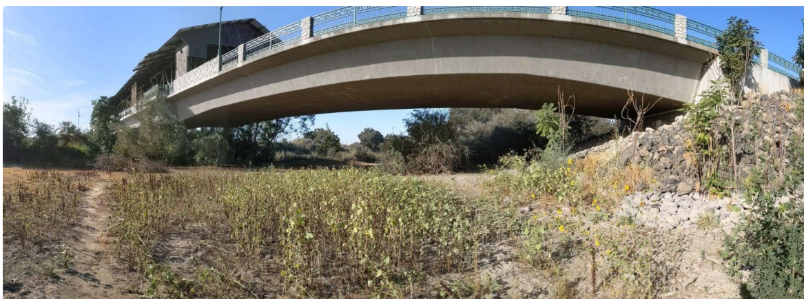
Figure 16. Photo of the overbank area under Robert's Ferry bridge taken on October 13, 2023 at a flow of 1,000 cfs. The geometry of the bridge (e.g., the span, height, location of pylons) is not expected to present any issues in terms of large woody debris racking.
