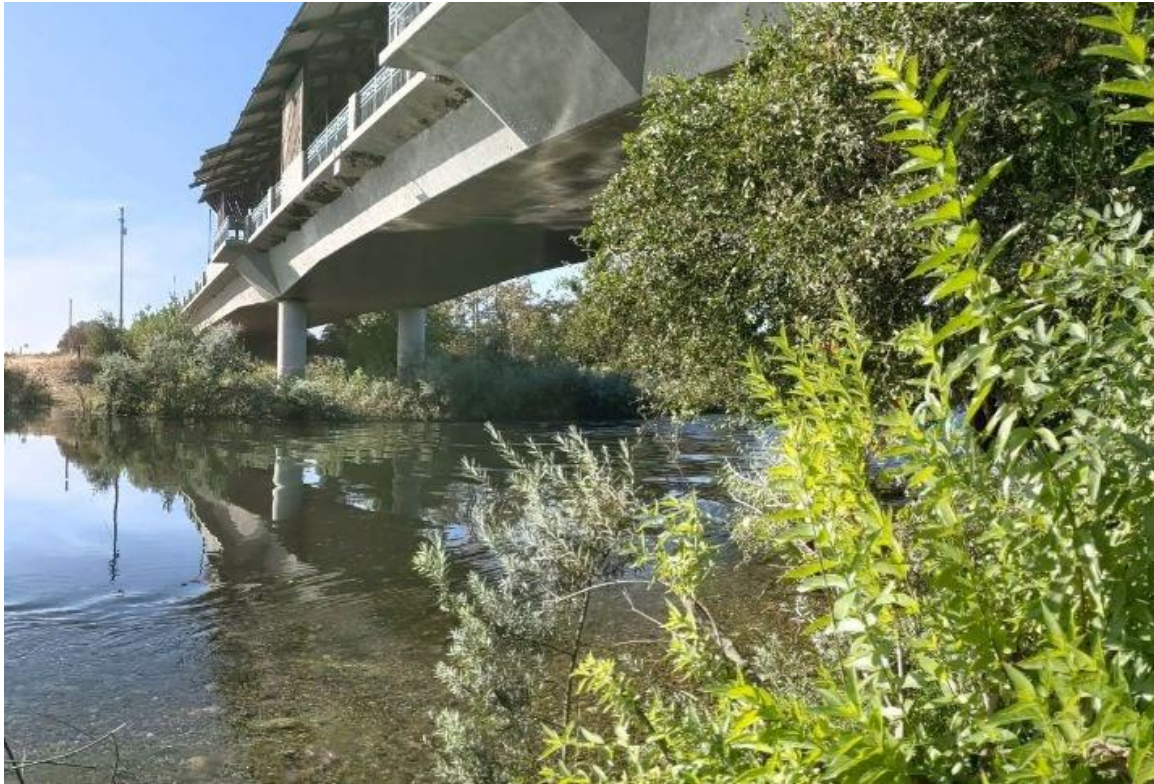
Figure 15. Photo of the Tuolumne River channel under Robert's Ferry bridge taken on October 13, 2023 at a flow of 1,000 cfs. The geometry of the bridge (e.g., the span, height, location of pylons) is not expected to present any issues in terms of large woody debris racking.
